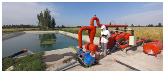
Fig. 4. Filter station in research polygon
